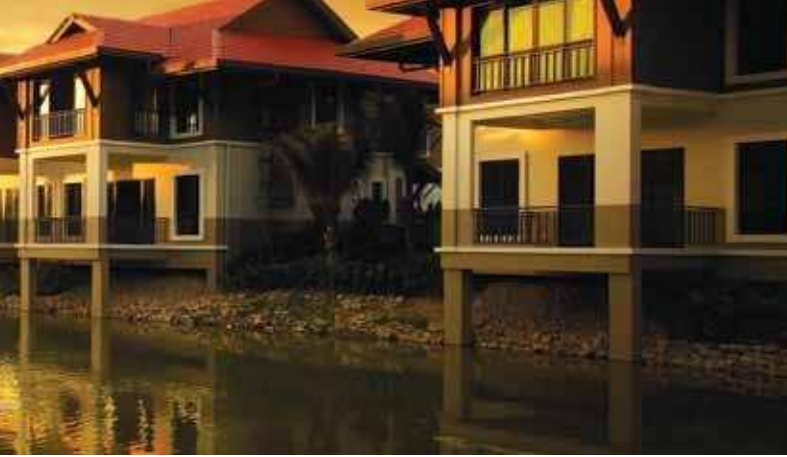
Bayou Water Village comprised of bungalows, semi-detached and terraced homes overlooking the canal.
